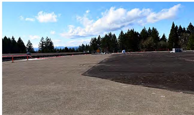
Protective coating being added to the roof of Fernhill Reservoir #1.
