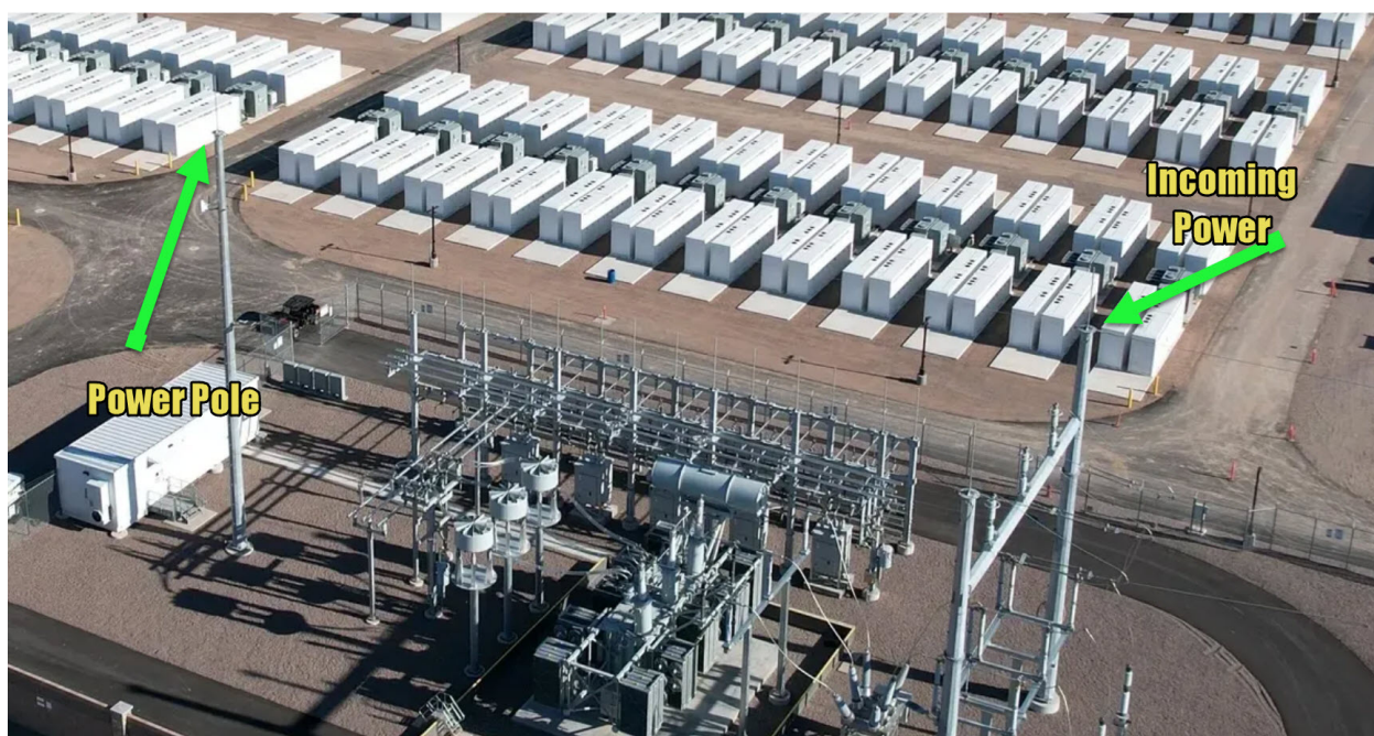
Photo 5: Photo of BESS Battery with Associated Power Pole & Connections
