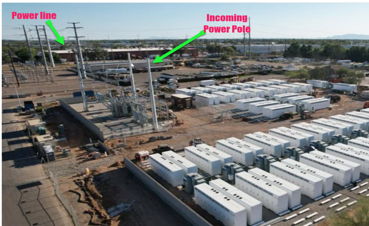
Photo 4: Photo of BESS Battery with Associated Power Pole & Connections
