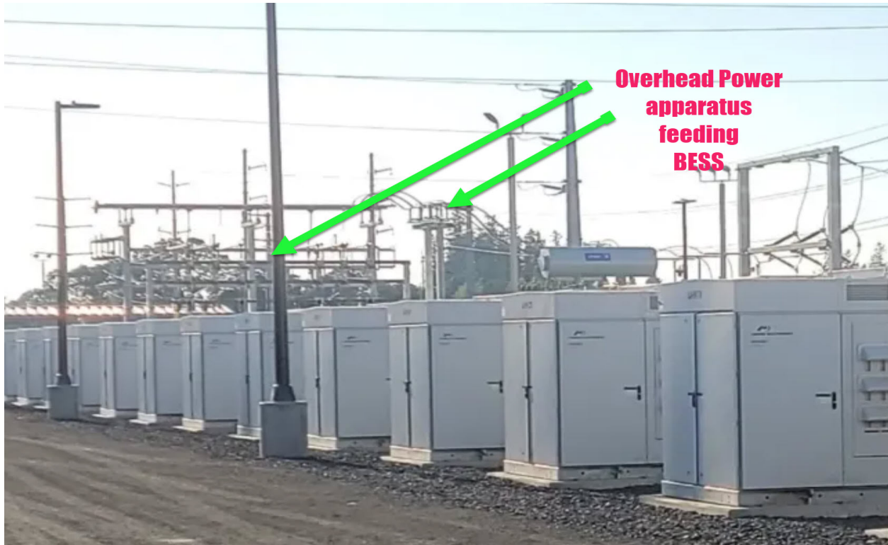
Photo 3: Photo of BESS Battery with Associated Power Pole & Connections
