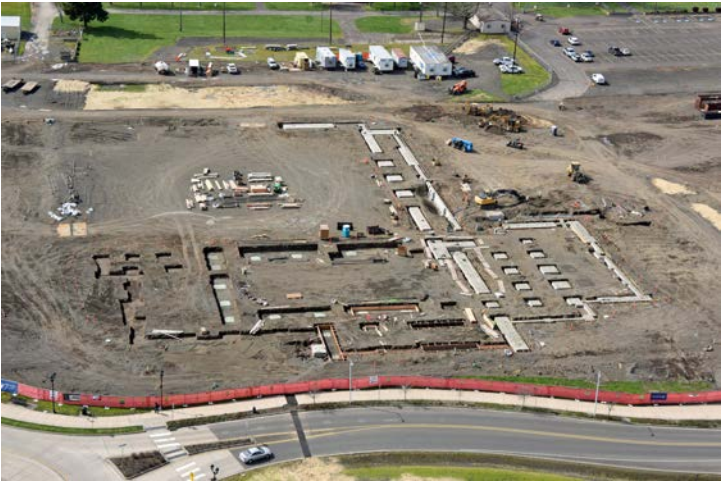
-Footings poured and building footprint takes shape. Area A shown to right, Area B adjacent to NE 34th Ave.
