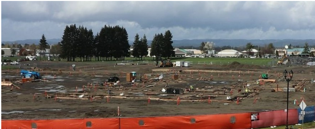
-Foundation work at the site during the spring dry weather
