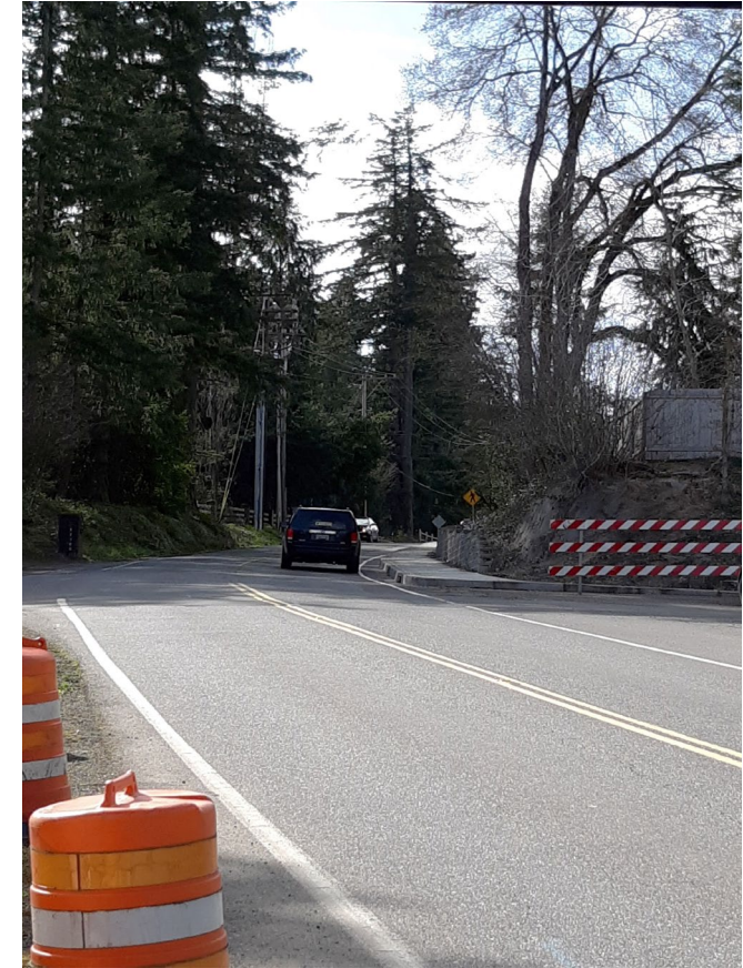
URMD Interim Sidewalk (Phase 4)
