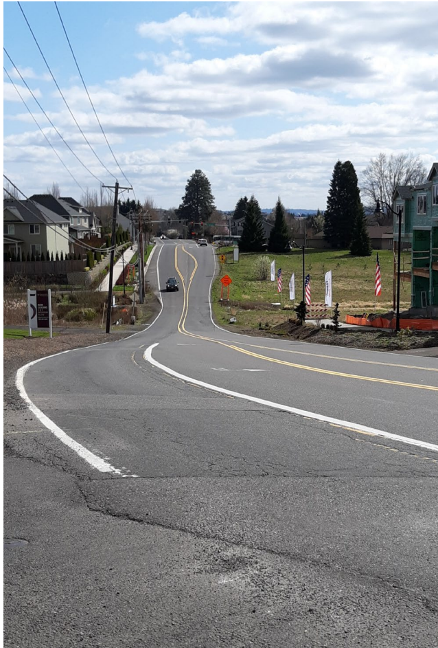
Looking south from Brugger Road
