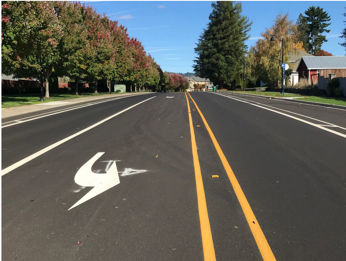
At Joss Avenue looking east
