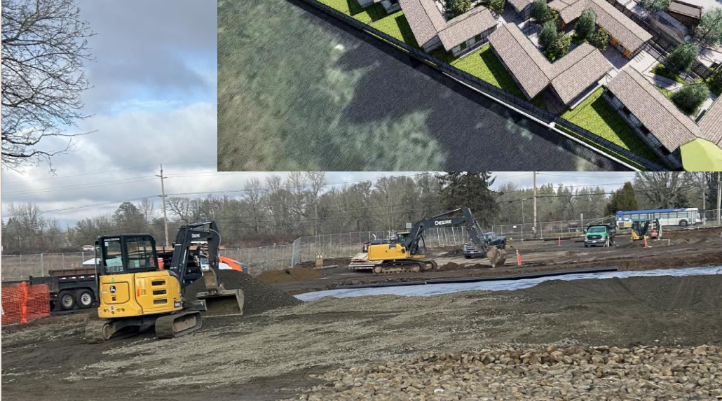
Hillsboro Shelter rendering and construction site
