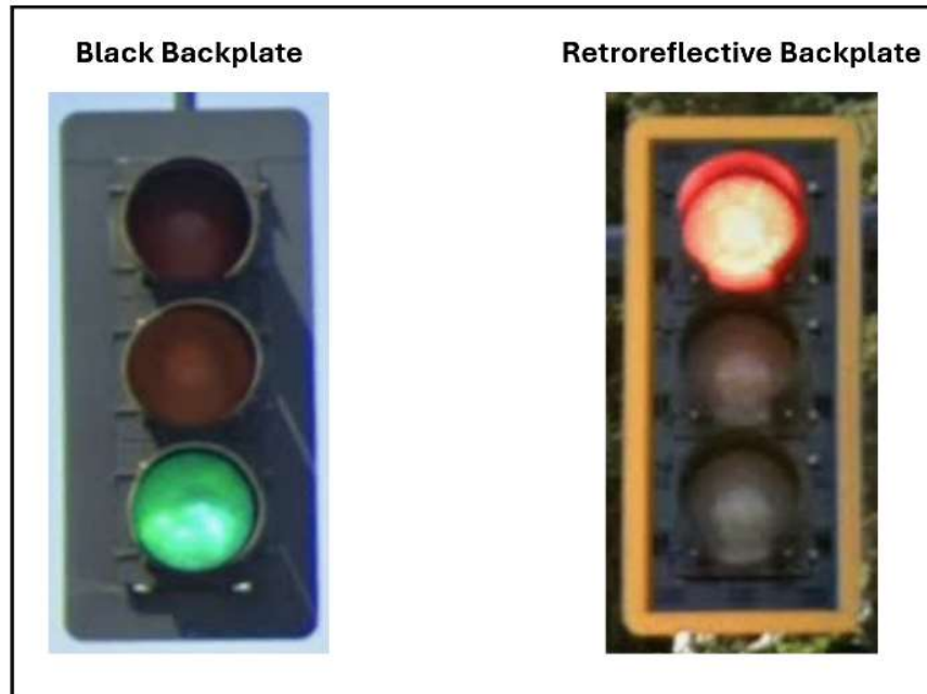
Figure 1: Typical example of signal heads with black backplates (left) and retroreflective backplates (right). Figure 1: Typical example of signal heads with black backplates (left) and retroreflective backplates (right).
