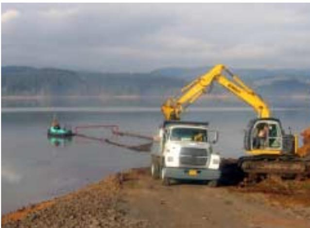
Debris is pushed from dam face into V-trap (top), delivered to shore and then removed (bottom).
