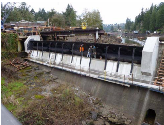
Left: Lake Oswego Dam spillway after modification with gates are in raised position during installation of the restraining straps. Air bladders are visible behind straps.
