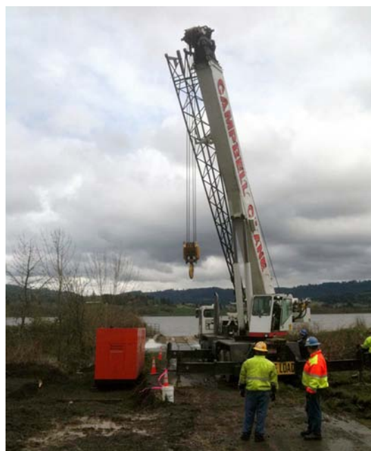
Crane lifting large BES pump.
