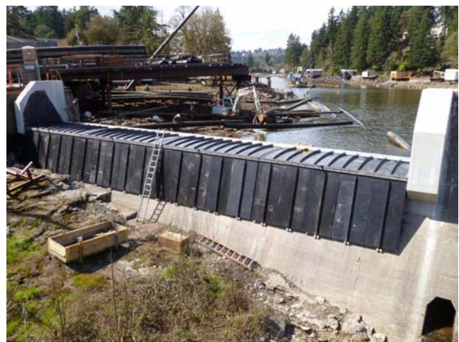
Left: Lake Oswego Dam spillway after modification with gates are in raised position during installation of the restraining straps. Air bladders are visible behind straps.
