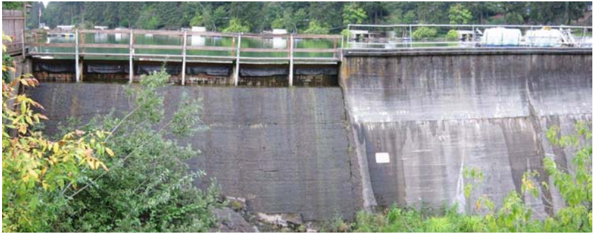
Lake Oswego Dam spillway before modification.
