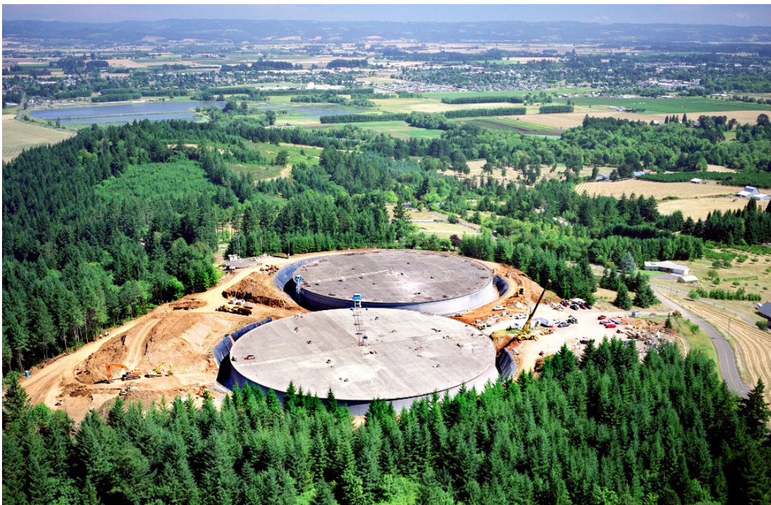
Each Fern Hill Reservoir stores 20 million gallons of drinking water for the Joint Water Commission.
