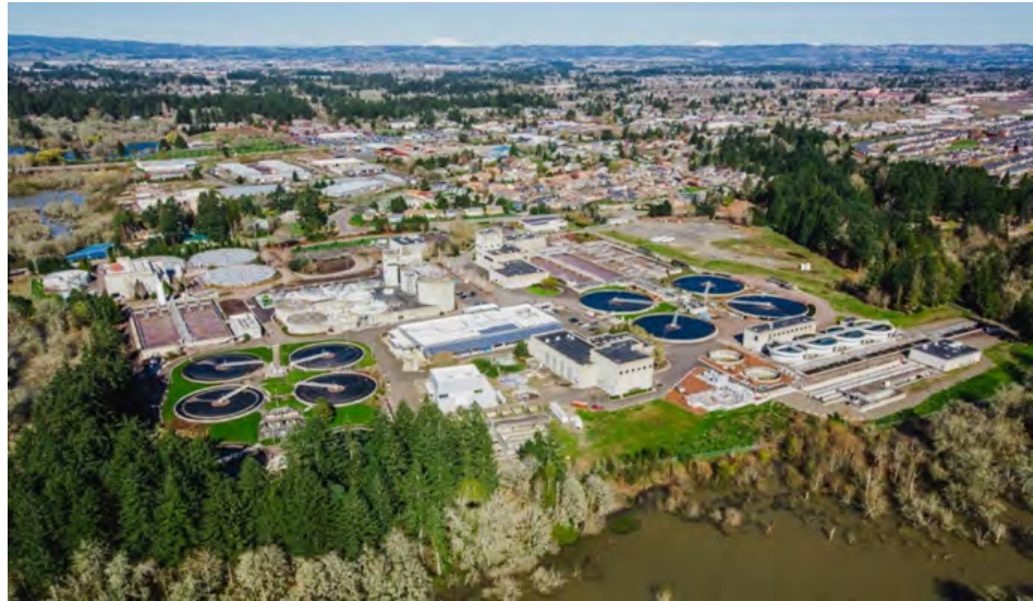
Rock Creek Wastewater Treatment Facility
