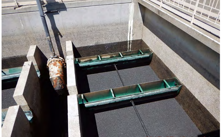
New sand and anthracite media installed in the filters
