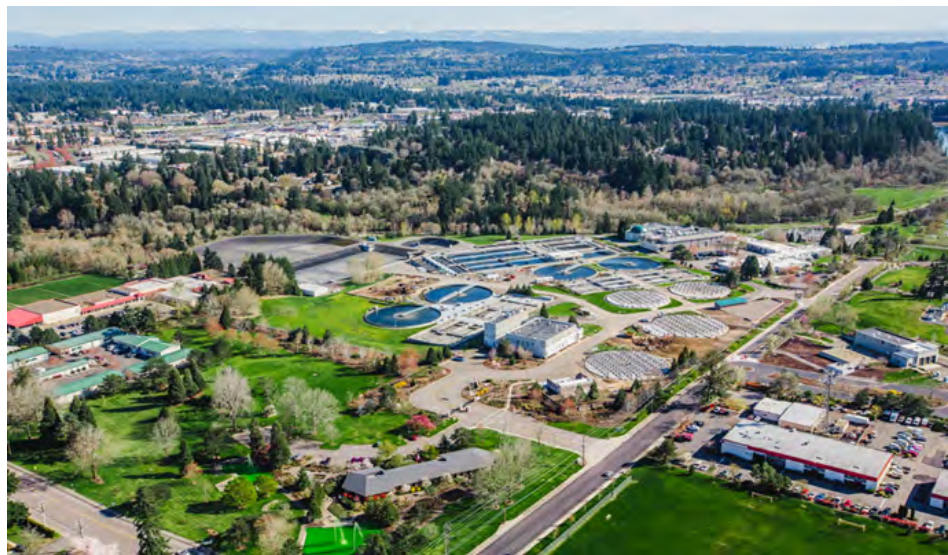
Durham Wastewater Treatment Facility
