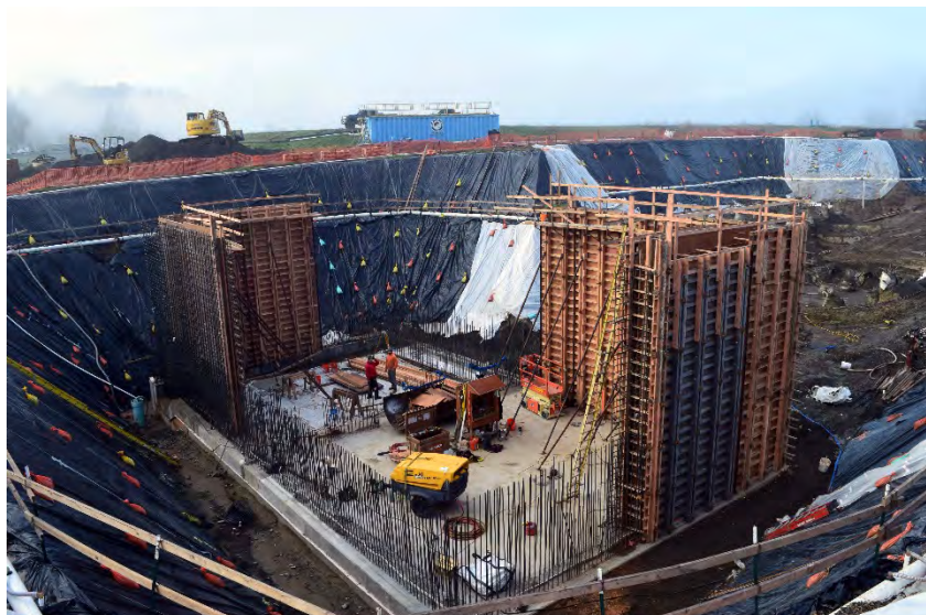
Concrete slab completed and concrete walls in progress
