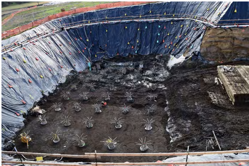
Auger cast piles installed for forthcoming concrete structures
