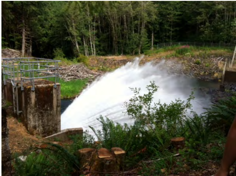
Release from Barney Reservoir to the Trask River through a Howell-Bunger Valve
