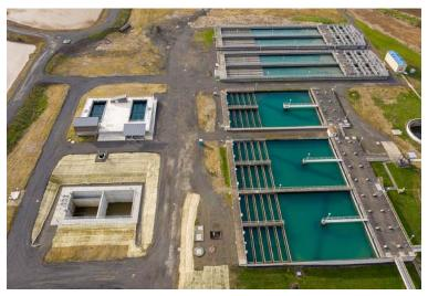
New filters (top left) and surge basin (bottom left) were constructed near the existing sedimentation basins at the JWC water treatment plant to expand capacity from 75 to 85 MGD.
